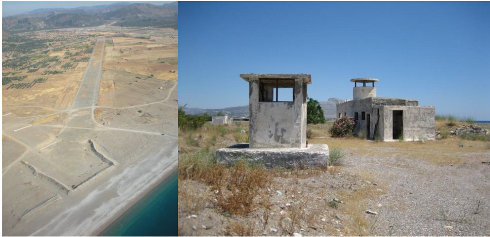
Airfield, and control tower
